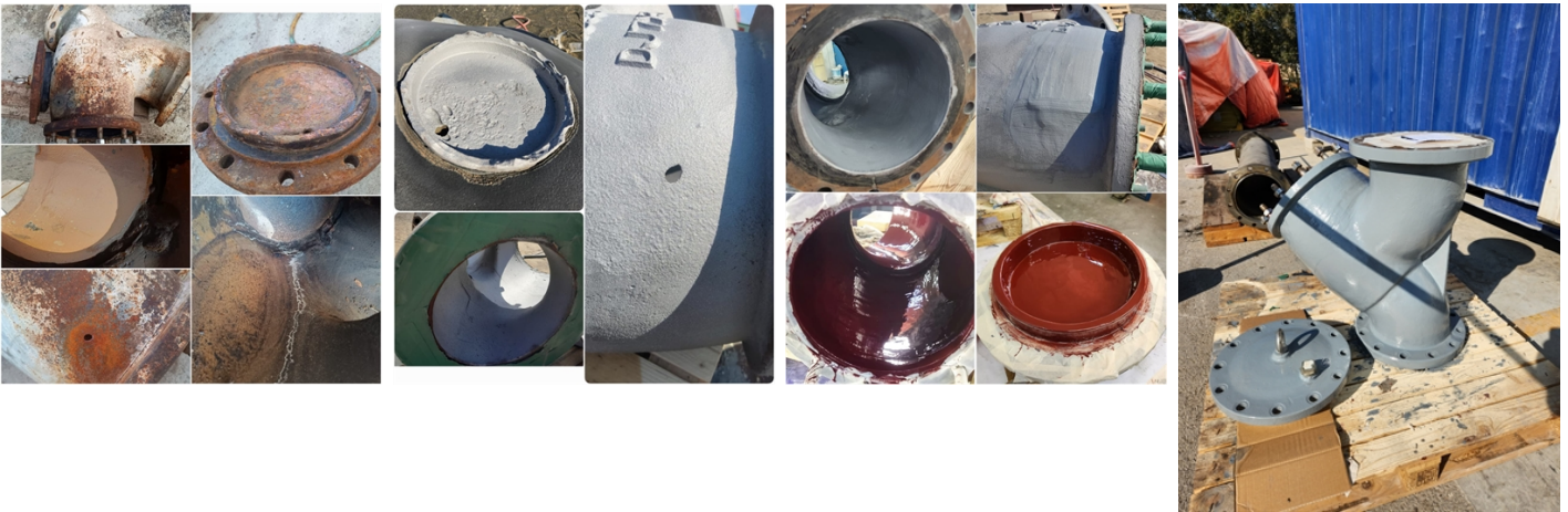
Initial condition of strainer
