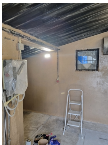
Coating of walls with Belzona 5811.
