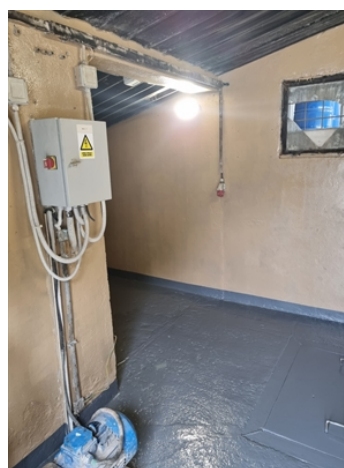
Application finished on both walls and floor.
