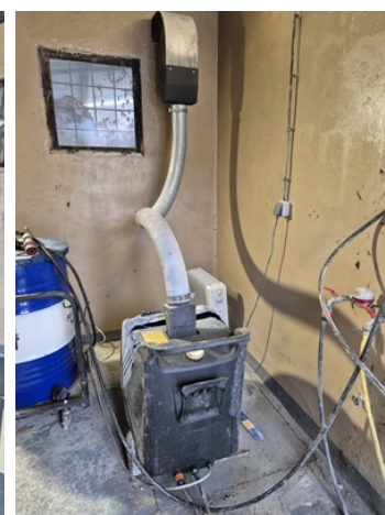
Situation after 2,5 years – coatings are still in good condition.
