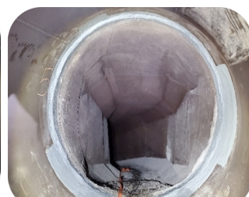
Final coating using a two-coat system of Belzona 5811 (Immersion Grade)
