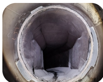
Damaged surface was rebuilt with Belzona 1111 (Super Metal) and Belzona 4131 (Magma-Screed)
