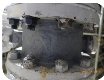
Belzona 1111 (Super Metal) applied on top of the emergency leak repair
