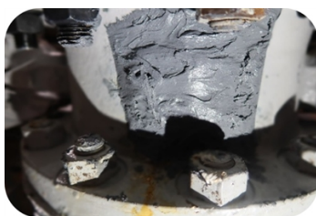
Belzona paste-grade materials, suitable for emergency repair, seal the leak on the valve
