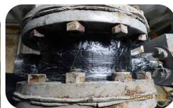
Belzona SuperWrap II was applied to reinforce the leak repair on the valve
