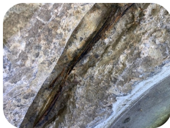
Surface preparation by a power
