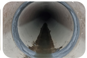
Belzona 5831 (ST-Barrier) coated flange surface subject to wet conditions
