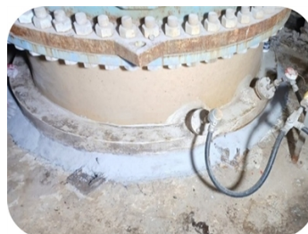
Belzona 4111 (Magma-Quartz) rebuilt the damaged concrete at the lower section of the condenser waterbox outlet
