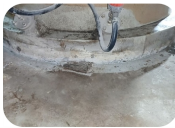
Surface preparation before rebuilding the damaged concrete
