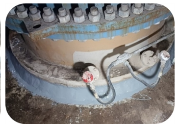
Belzona 5811 (Immersion Grade) coated on the rebuilt concrete at the lower section of the condenser waterbox outlet
