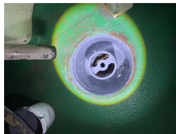
Two coats of Belzona 5831 (ST-Barrier)
