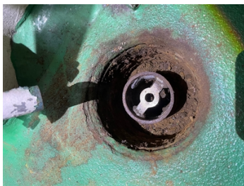
The original condition of the scupper
