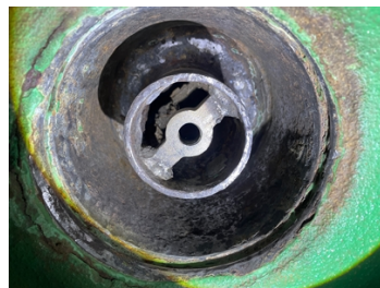
After surface preparation with a power file
