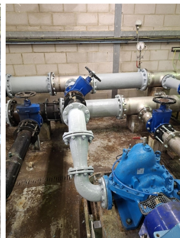
Pipework successfully protected with a corrosion-resistant coating, ensuring long-term durability
