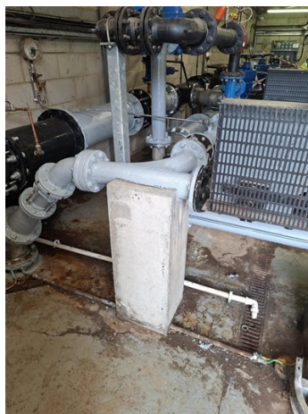
Completed application of protective coating system, restoring and protecting the pipework
