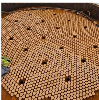
Corks fitted and ready for Grit Blasting, prior to filling with Belzona 1511
