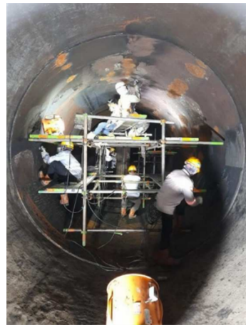
Rubber lining was removed before the application of a more permanent abrasion and erosion resistant system
