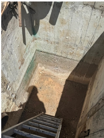
original condition of pit
