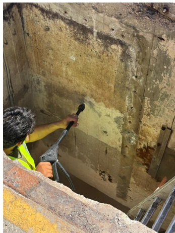
During surface preparation
