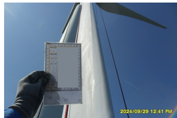
Belzona 5711 rebuilt a wind turbine leading edge
