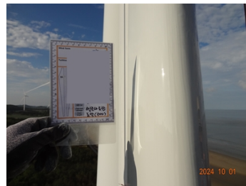
Belzona 5721 was applied as a single-layer coating on a wind turbine leading edge
