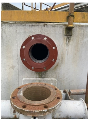
Flange rebuilt with Belzona 4301
