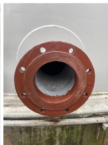
Flange rebuilt with Belzona 4301
