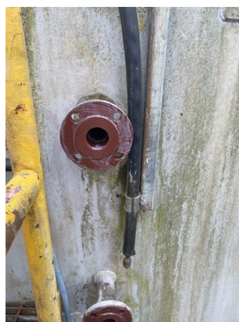
Flange rebuilt with Belzona 4301
