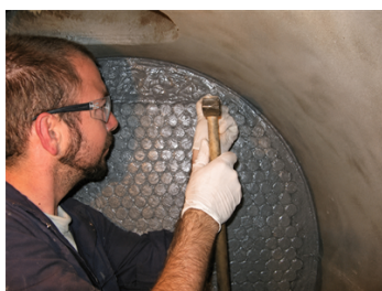
Protection of Belzona 1321 on heat exchanger
