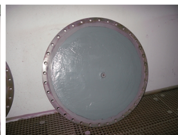
Finished application of Belzona 1321 on heat exchanger end cover
