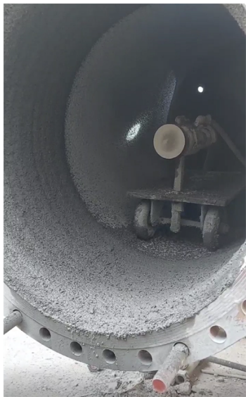
Shotcrete was applied centrifugally to the internal surface of slurry pipeline
