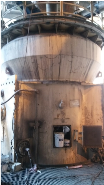
Application of Belzona system in a confined space
