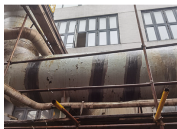
Application of Belzona Superwrap II
