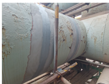
Application of Belzona 1212 and Belzona 1111
