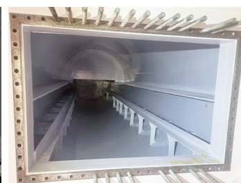
Final application of Belzona 1523 applied to the intercoolers.
