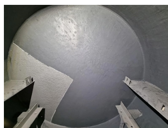
Pit filling and metal repairs undertaken with Belzona 1511.
