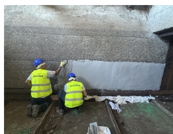
Application of Belzona 4111 (Magma-Quartz).
