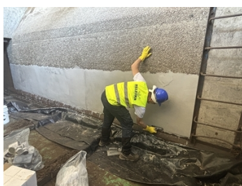
Application of Belzona 4111 (Magma-Quartz).
