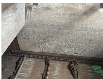
Condition of the structure prior to the repair work.
