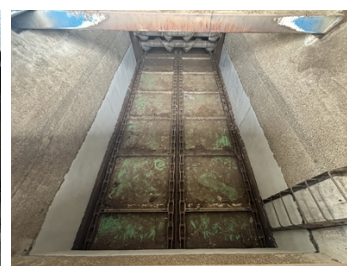
Work successfully completed.
