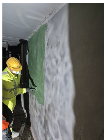
Belzona 1813 application in progress
