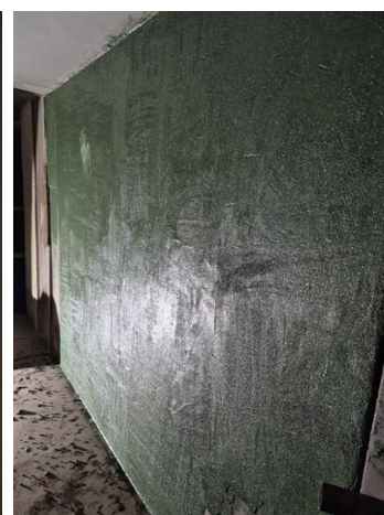
One affected area after Belzona 1813 application.
