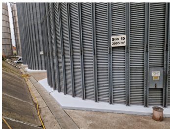
All tank foundations repaired and protected with Belzona 3111
