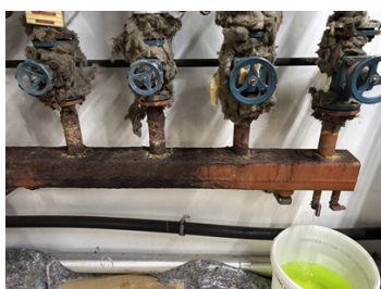
Corroded manifold
