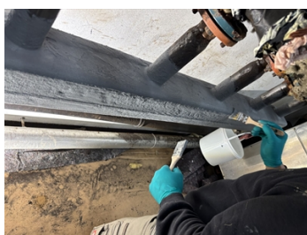
Substrate repaired using Belzona paste-grade materials
