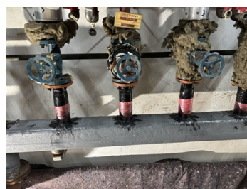
Start of the Super Wrap II application
