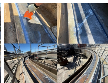
Filled bolt holes and completed repair
