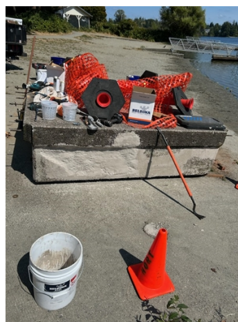
Floating dock during application.
