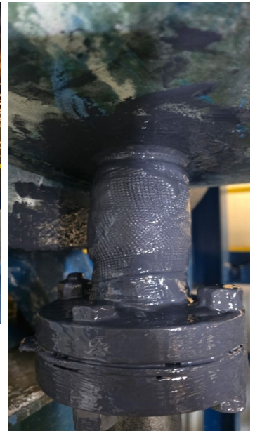
Application complete with multiple wraps of Belzona 9341 reinforcement sheet and Belzona 4311.
