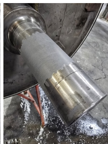
Former removed and the Belzona 1111 refined to the proper profile.
