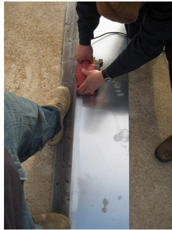
Preparing the panels
