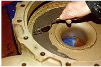
Belzona® 1311 being applied into the rebate at the extremity of the repair
