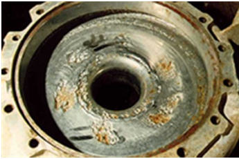
Typical casing showing the general erosion damage
