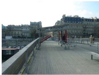
Non-disruptive application in 2000
