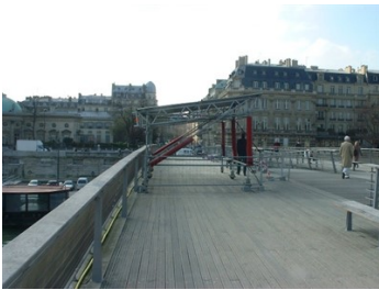
Non-disruptive application in 2000
