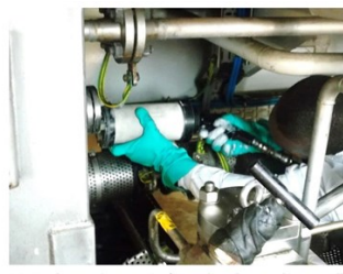
Injecting Belzona Compound to fill Any Gaps Between Plates and Tank
