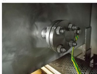
Surface Area Ready for Belzona and Metal Plates
