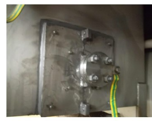
Plates and Belzona Applied to Affected Area; Reading for 2 Hour Curing
