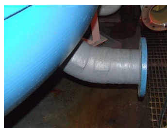
Plate bond &amp; wrap applied
