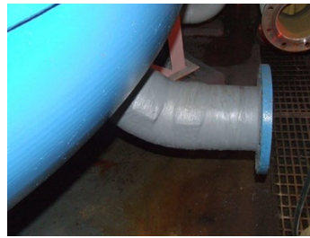
Plate bond &amp; wrap applied
