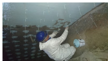
The first layer of Belzona 1593 product.
