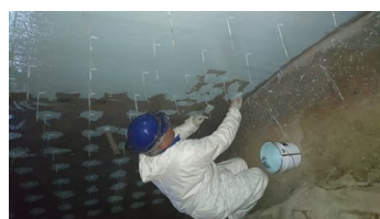
The first layer of Belzona 1593 product.
