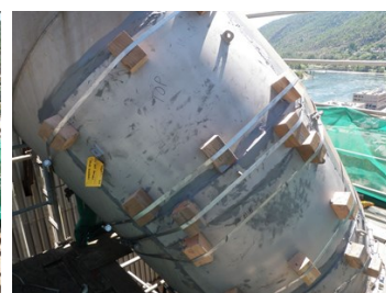
All 5 plates bonded in place; application is completed
