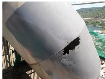
Prepared area coated with Belzona 5841
