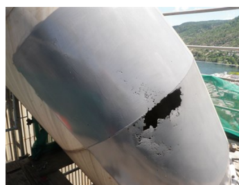
Prepared area coated with Belzona 5841
