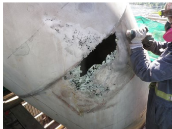
Initial surface preparation using a wire brush
