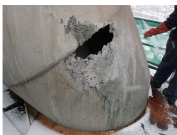
View of small holes indicating extensive pitting of the interior surface
