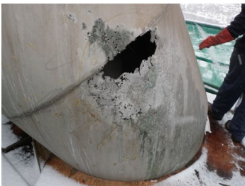
View of small holes indicating extensive pitting of the interior surface
