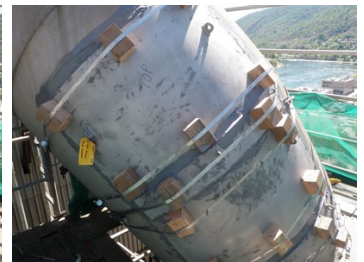
All 5 plates bonded in place; application is completed
