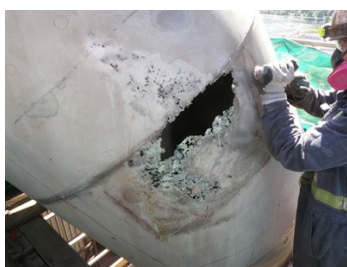
Initial surface preparation using a wire brush
