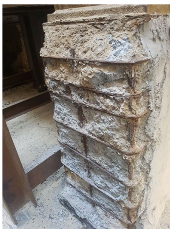
Damaged and loosely adhered concrete removed
