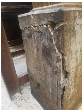
Cracked and Spalling Concrete
