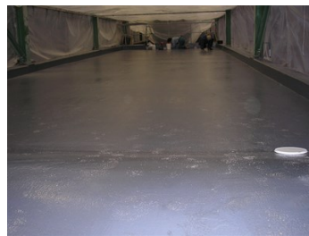
Belzona 4311 after being applied
