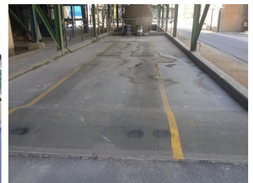
Wear pads and flooring system 8 years later
