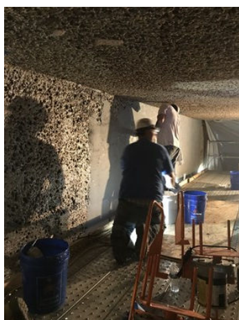
Rebuilding concrete with 4131
