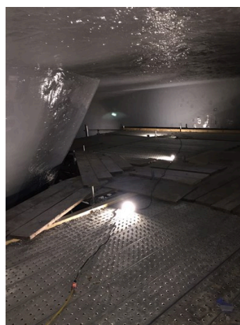
Tunnel coated with 5811
