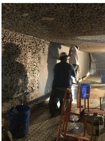
Rebuilding concrete with 4131
