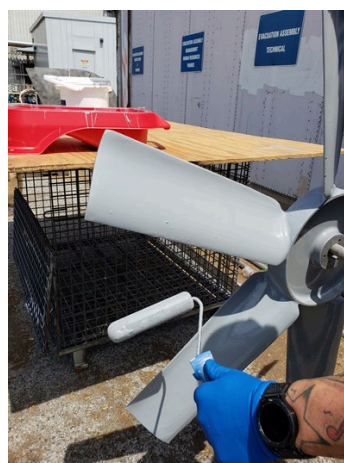
Fan being coated
