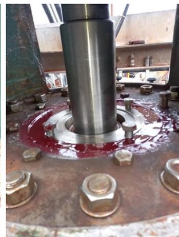
Belzona 4331 filled to replace the lost metal
