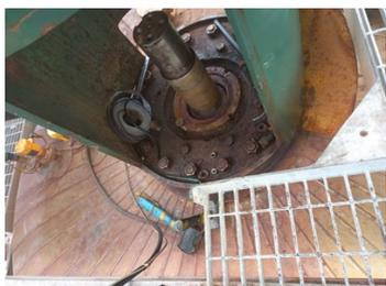
Corroded area around mechanical seal
