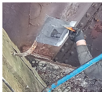
Belzona 1121 plate bonding
