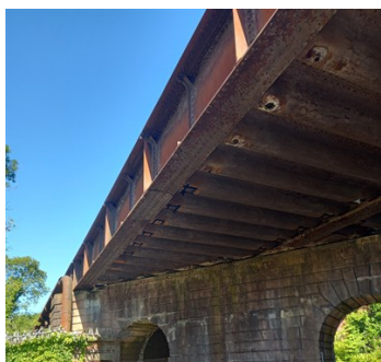
Bridge with leaking sections
