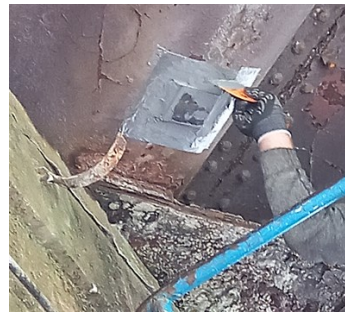
Belzona 1121 plate bonding
