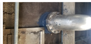
Finished application (far angle).
