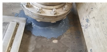
Finished application (close angle).
