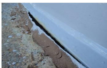
Original mastic failure
