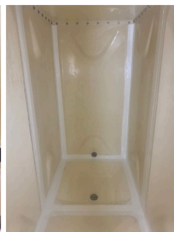
Belzona 5811DW2 applied as a top coat
