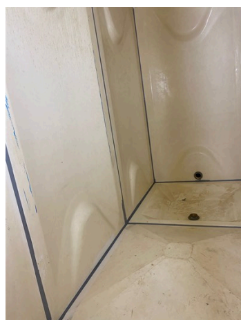
Belzona 1111 applied to fair the gaps between the tank sections
