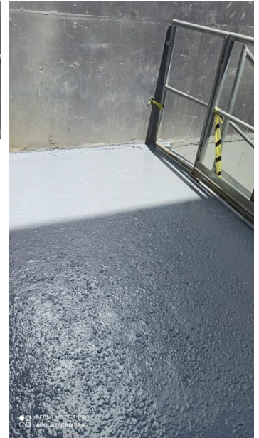
Accessing floor also coated
