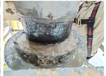
Hole repaired with SuperWrap II.
