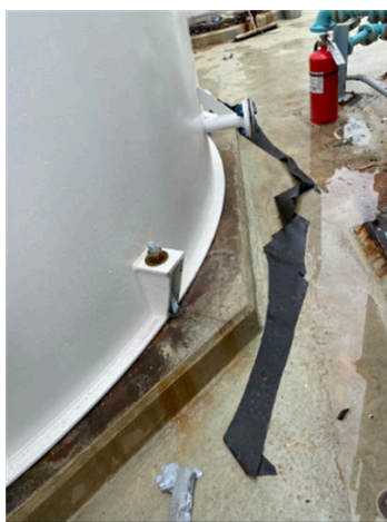
Previous coating was removed.
