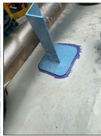
Belzona 7311 to bond pipe supports to the top of the tank.
