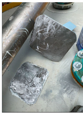
Areas on top of the tank prepared with a Bristle Blaster to remove paint.
