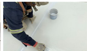
Final coat being applied.
