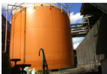
Photo of the tank
