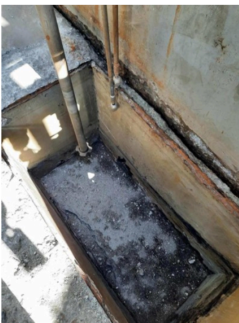
Damage to the sump pit area.
