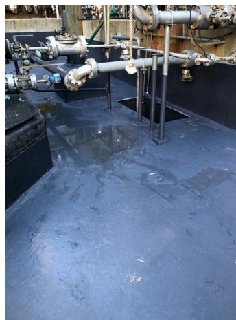
Finished repair and coating. Belzona 4311 was used.
