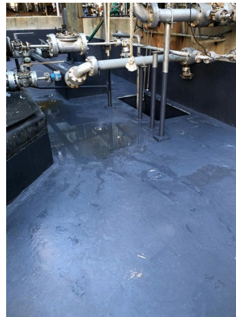
Finished repair and coating. Belzona 4311 was used.
