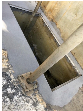
Repairs that were made using Belzona 41111.
