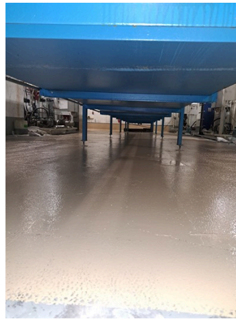
Final coat of Belzona 5831 (ST-Barrier) being applied to all accessible areas
