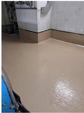
Belzona 4111 (Magma-Quartz) was used to build a cove at the joints with the perimeter walls, and overcoated with Belzona 5831 (ST-Barrier)
