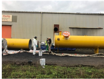
Pipework mid-application of Belzona 5811.
