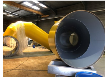
Finished internal & external lining application using Belzona 5811.
