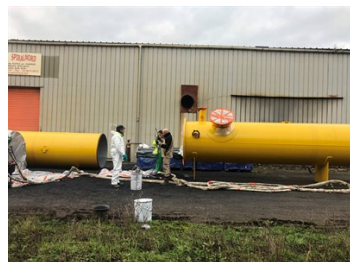
Pipework mid-application of Belzona 5811.
